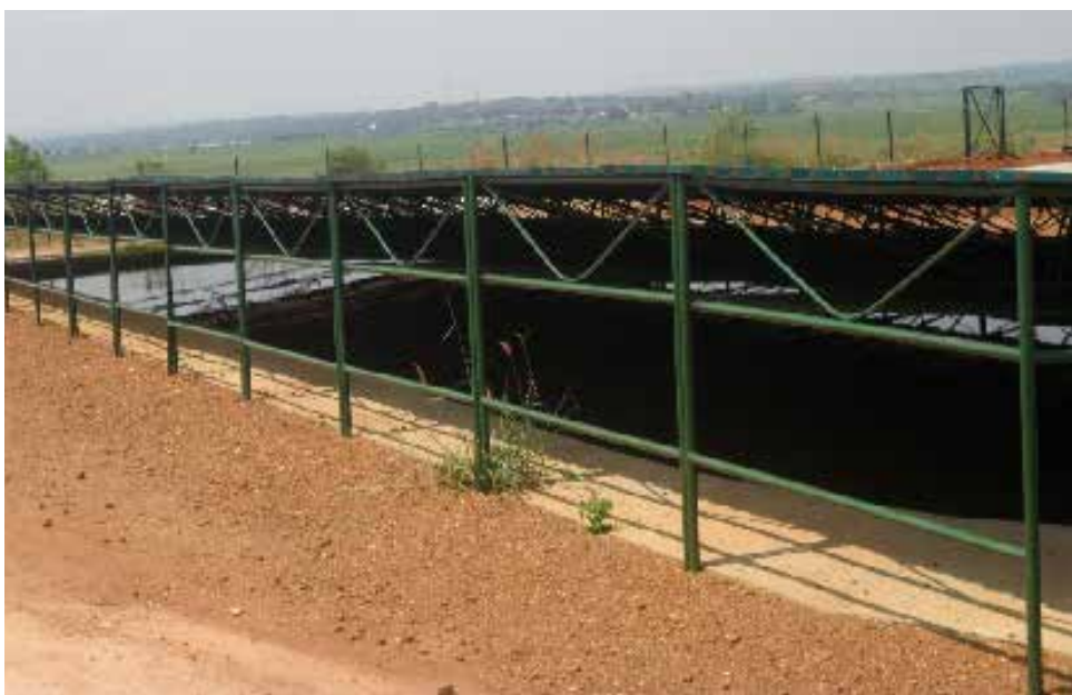
Liquid wastes were being stored in pits with slanting iron roofing .
